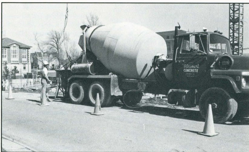
Pouring concrete (Tate Hall in background)
