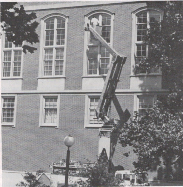
Weathered windows receive new paint
