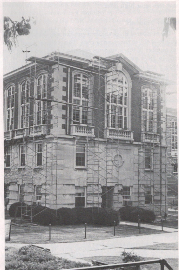
New guttering being installed
